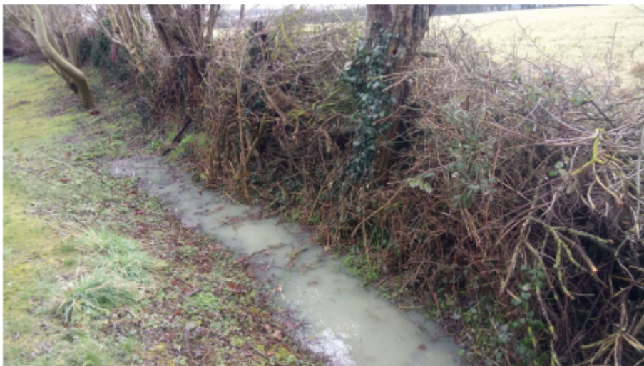
Photograph 3: Further evidence of flooding at 119 West Street, Helpston on its border with the proposed area for development in 17/01448/OUT, 10/03/2018
